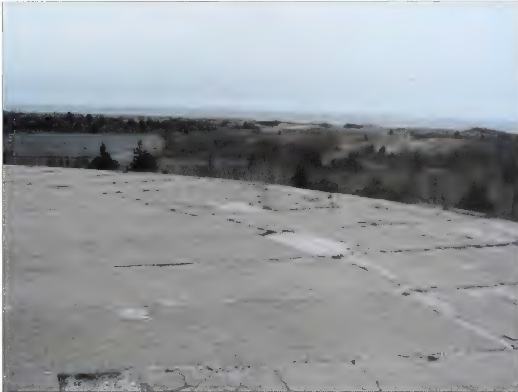
Figure 3.25. View looking northeast across superior slope, Battery Potter. On top of Battery Potter, the superior slope proceeds east from the terreplein that contained two openings for raising and lowering the 12-inch caliber guns (Olmsted Center, April 2008).
